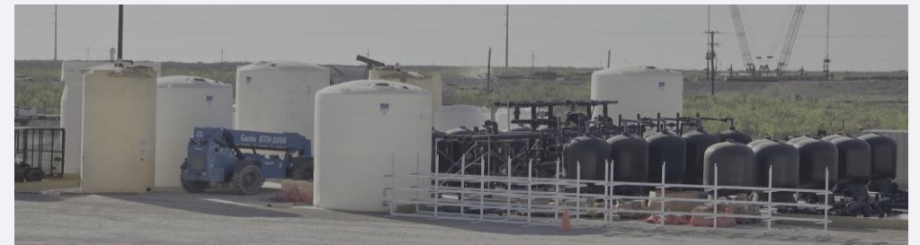
Element3 33,000 BWPD plant in installation
